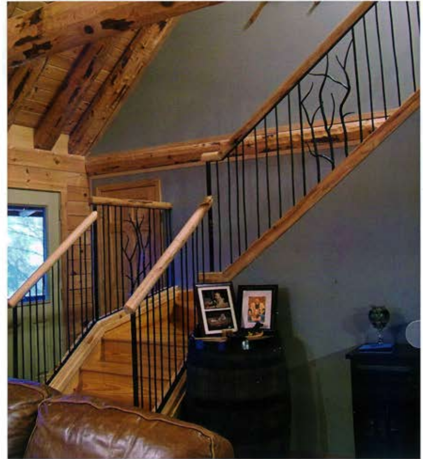
Rustic Railing. The new railing was designed to take advantage of existing carpentry, using the same wood curb rail to anchor the new steel balustrade. A collaborating carpenter matched the log construction with a wood handrail fastened to a top channel, further simplifying construction and installation of the steel.
